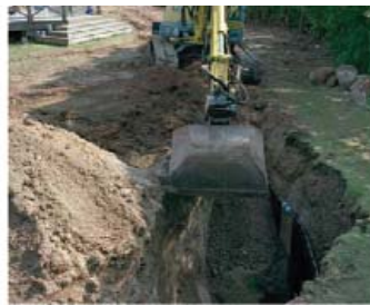
The trench is refilled.
