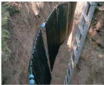
The sections are easily connected together at the top.
